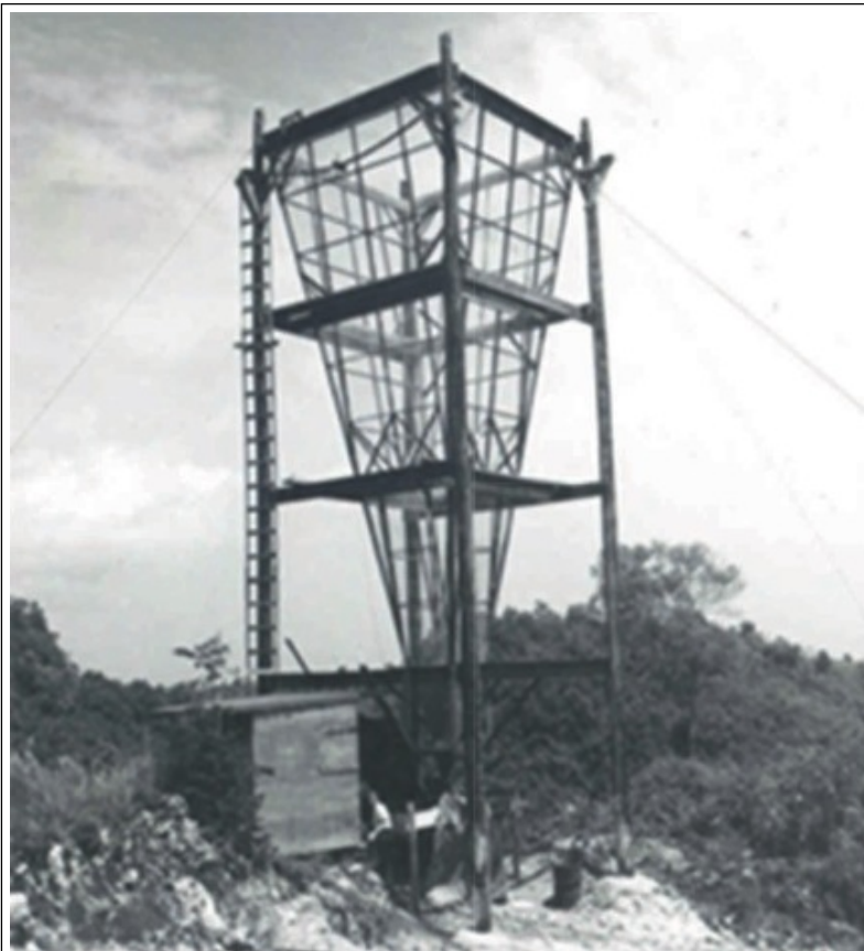
Figure 1. The first functioning radar feed at AIO. This 430 MHz hornfeed was constructed to test the full radar system before the dish was completed. This feed had a \sim 10^\circ half-power beamwidth and was in operation in mid-October 1962. It was used to receive the sun in transit and to obtain lunar echoes as the moon transited near zenith [Gordon, 1962]. Photo courtesy of Carmen G. Segarra-Saavedra [Mathews, 2013b; Segarra-Saavedra, 2012]. Figure 4, [Mathews, 2013a].
